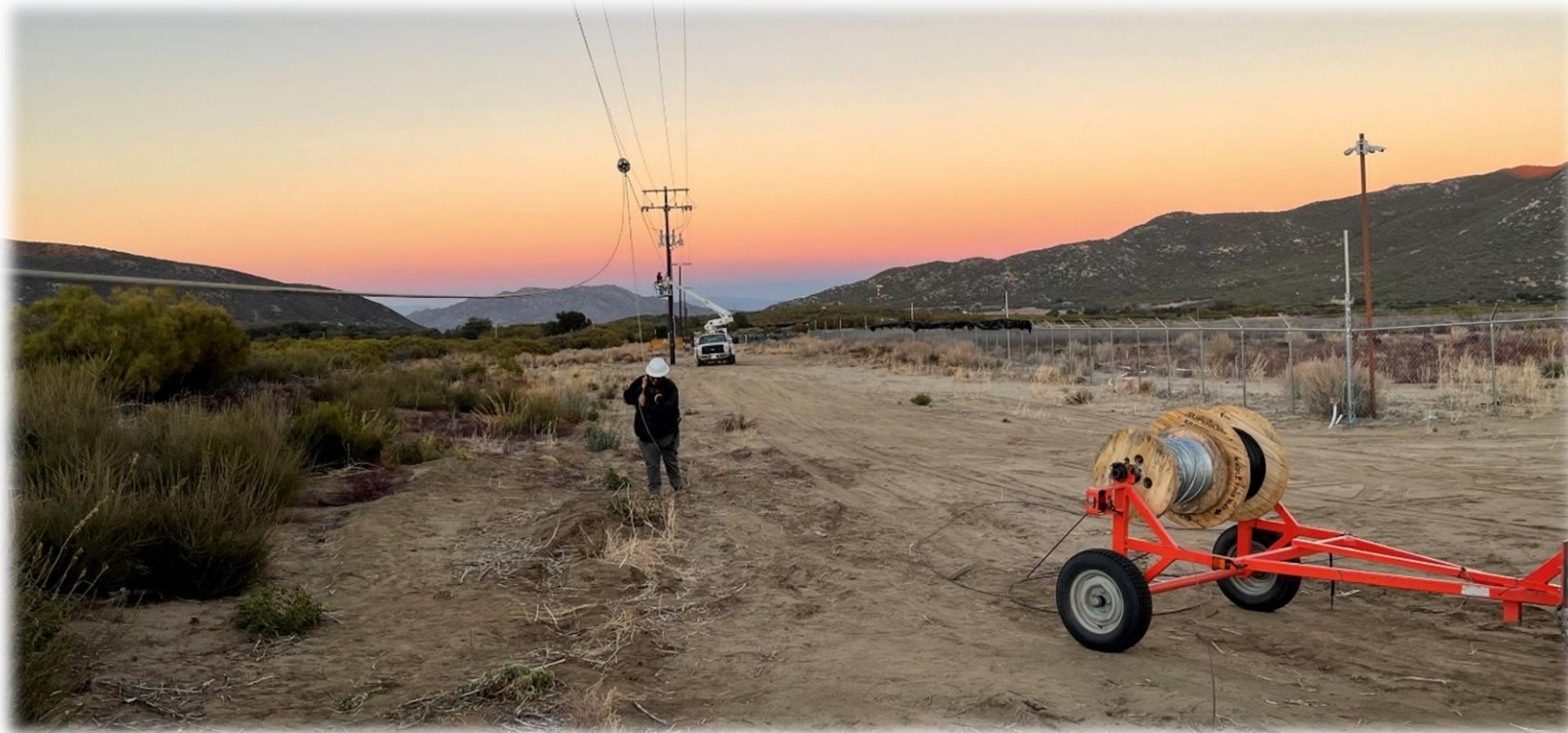
Deployment of Anza Electric's CASF Connect Anza project, Riverside County
