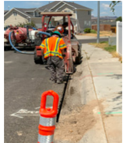
Figure 3: Example of a microtrench in a residential neighborhood
